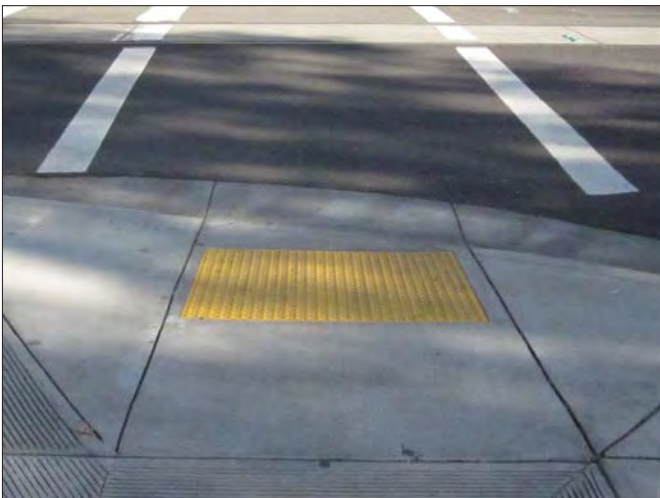
Tuncated domes alert the sight-impaired to roadway crossings. Typically yellow to contrast with concrete walkways, they can be other colors as long as they provide sufficient contrast with the surface.
