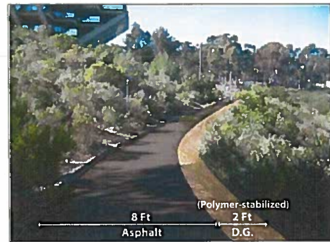
The path will be asphalt with polymer-stabilized decomposed granite on one side.
