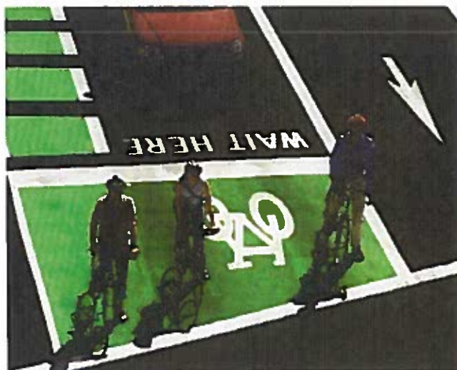
Bike boxes provide an advance stop position for cyclists to ensure their visibility to drivers and to encourage proper cyclist positioning when traveling straight through an intersection that allows vehicle turning.
