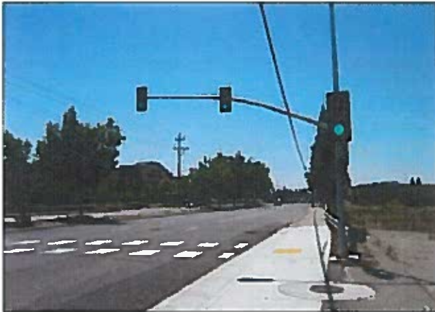
The traffic signal should have vehicle and pedestrian-controlling indicators and should be timed to prioritize pedestrian travel during class change periods.
