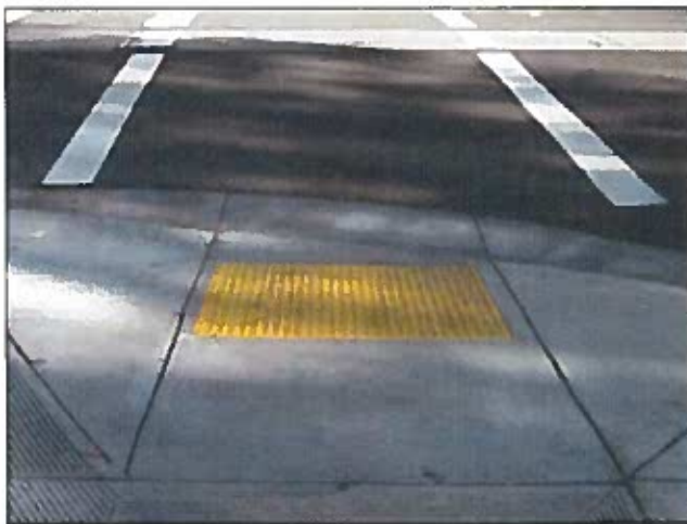
Tuncated domes alert the sight-impaired to roadway crossings. Typically yellow to contrast with concrete walkways, they can be other colors as long as they provide sufficient contrast with the surface.
