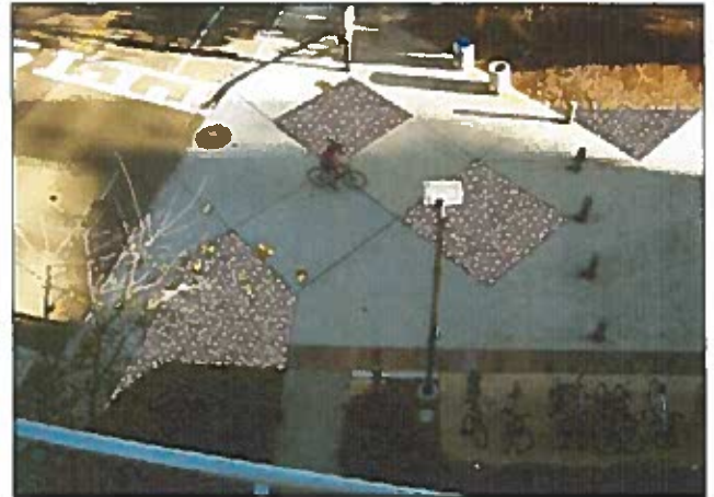
The chicane is intended to coordinate with the existing paving scoreline pattern. Specific concrete sections would be replaced with fixed-in-place cobble.
