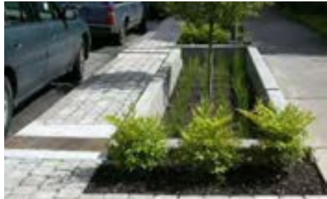
Flow through planters, located along streets, should be designed to accommodate all street and parking runoff and serve as a buffer between vehicles and pedestrians.
