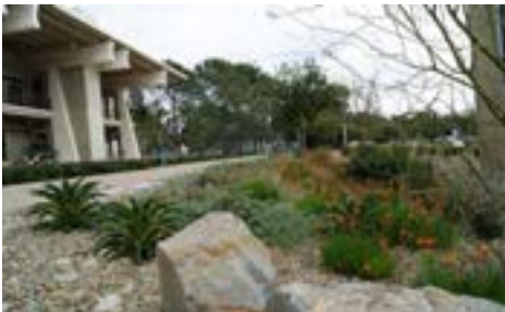
Bioretention areas should act as vegetated buffers along walkways and be designed to blend in with the adjacent landscape palette.
