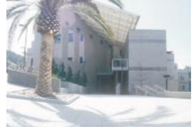
Ritter Replacement Facility entry plaza at the intersection of Discovery and Naga Way.
