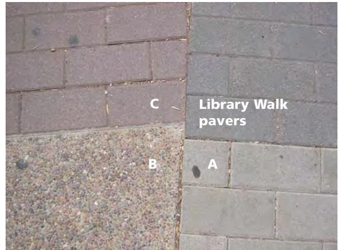
Figure 3-36 Pedestrian Pavement types
