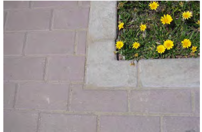
Figure 3-65 Detail of Russell Lane concrete pavers and header at the tree planting area
