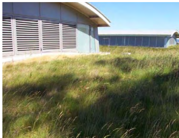
Green roofs can be used to counteract heat island effect
