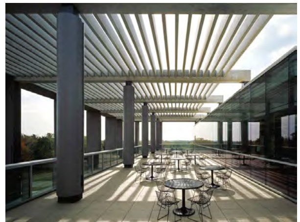
Usable outdoor roofs or balconies animate buildings
