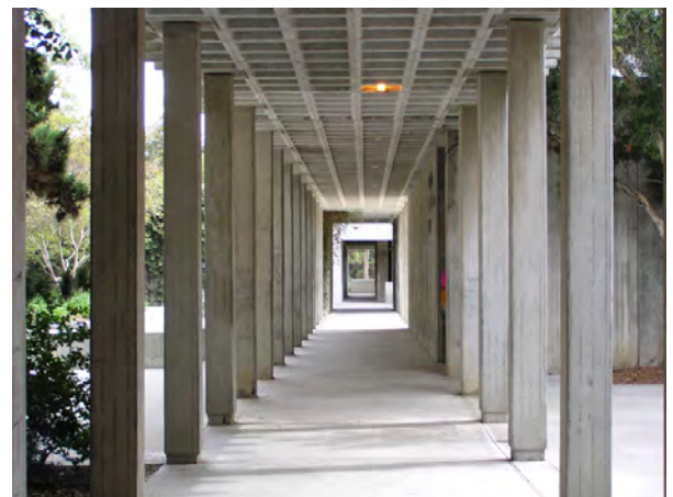
Shaded external circulation corridors and usable areas
