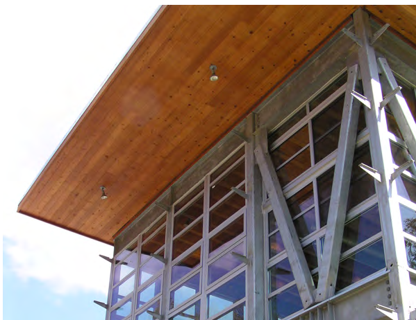
Roof overhangs for solar shading
