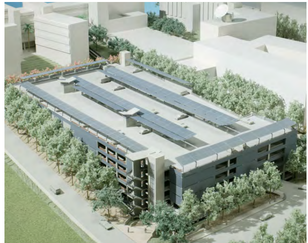
Parking structure utilizing photovoltaic panels for shade
