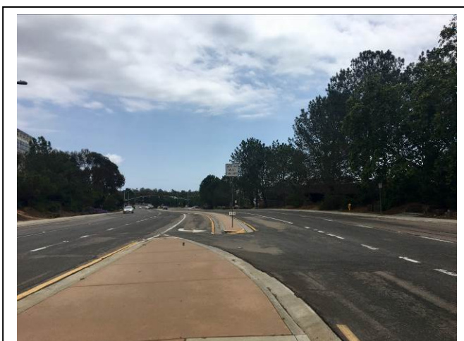
A traffic signal would be installed at the proposed fire station driveway intersection to allow fire apparatus to safely exit and enter the station. The median along North Torrey Pines Road (shown above) would be modified to prevent illegal left turns out of the Torrey Pines Center North driveway.
