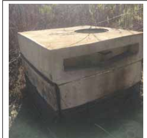
The existing drainage catch basin south of the project site is equipped with an overflow to restrict the volume and rate of runoff discharged from the basin.
