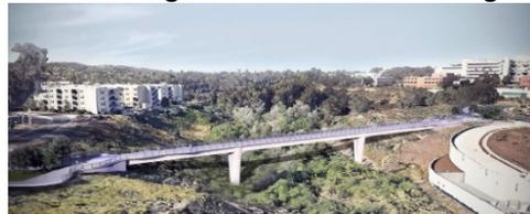
This bridge will provide a much-needed connection between Mesa Housing and the Medical Center. Spanning 465 linear feet, the bridge will feature a 10-foot-wide bike lane and a separate 6-foot-wide pedestrian walkway.
