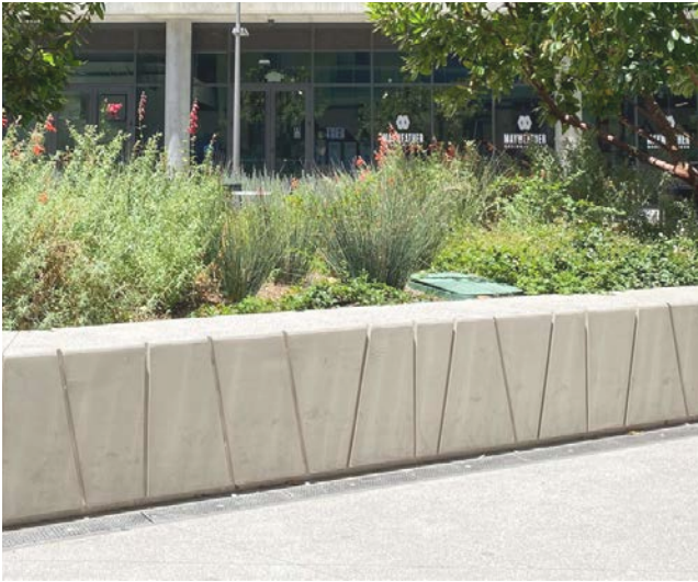
Precast Concrete Benches and CIP Concrete Pathway
